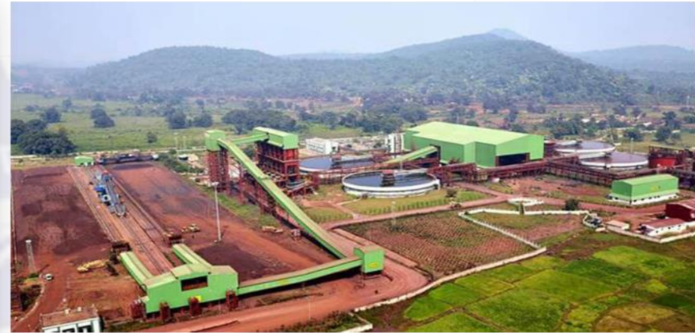
15 MTA Iron Ore Beneficiation Plant of Essar Steel at Barbil
