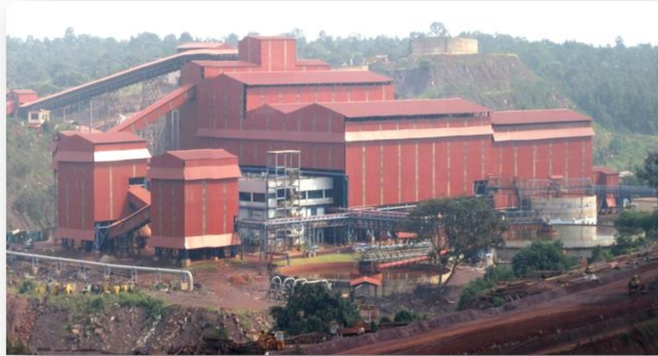
15 MTA Iron Ore Beneficiation Plant of SMPL at Barbil
